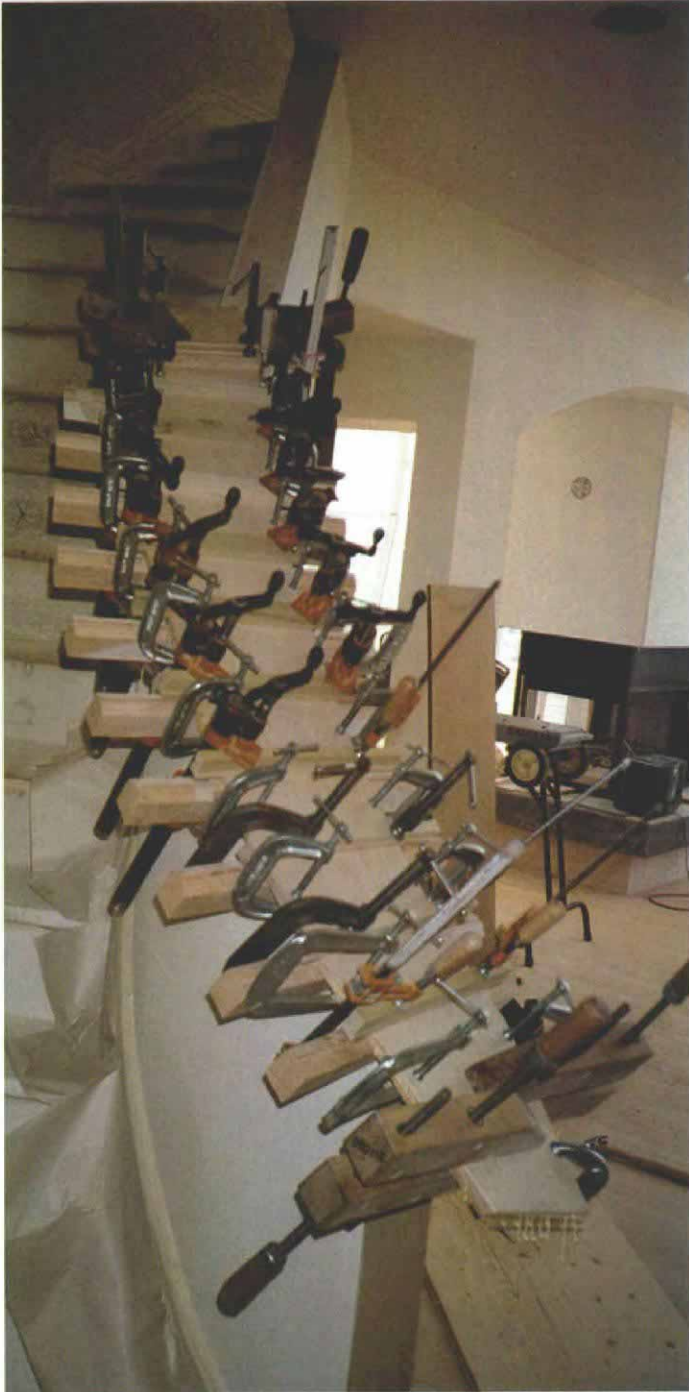
Gluing up. Even after the excess material was cut away, the maple proved to be so tough that only two layers could be glued at a time.
